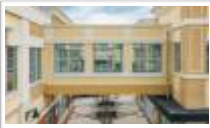
Bridge: Bridge at Stern & Eisenberg
