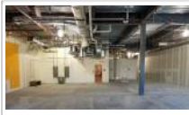
Non-Residential Building: Vanilla Box
